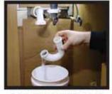
DUMP WATER AND REMOVE DEBRIS
