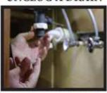
CLEAN WASHER, MAKE SURE TO RE-ATTACH WASHER WITH THE FLAT END UP
