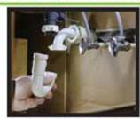
UNSCREW, & PULL APART. MAKE SURE YOU HAVE A BUCKET PLACED UNDER PIPES
